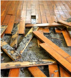
Leak Under The Floor
