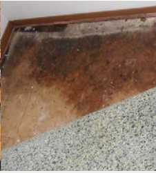
Leak Under The Floor
